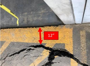
Note: It appears base has collapsed and void under pavement goes to foundation wall (6-12") and then slopes to bottom of hole.
