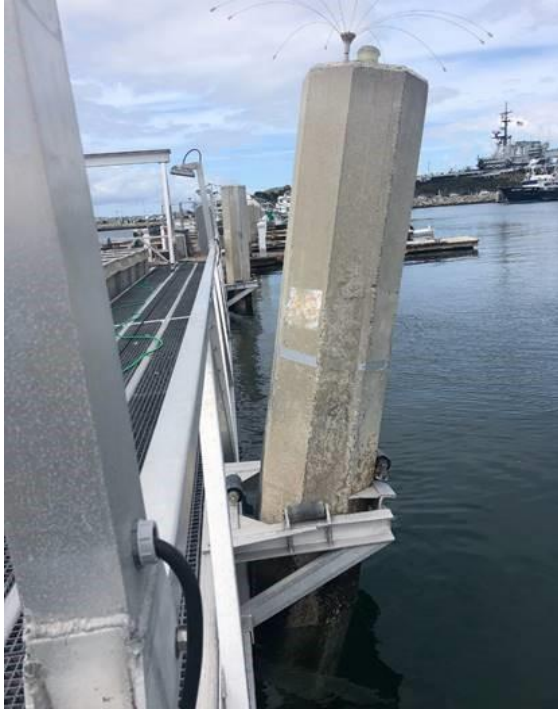
FLUPSY ATTACHED TO PILES
