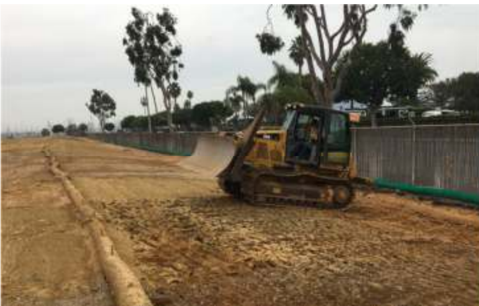
Best Management Practice (BMP) – Slope Tracking
