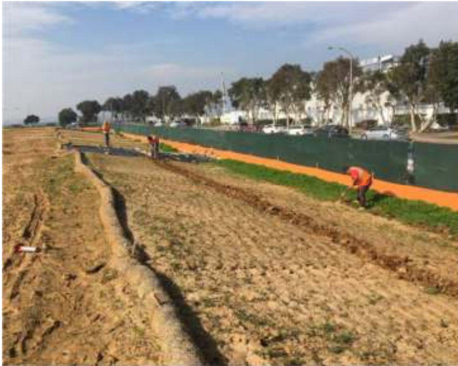
BMP Installation – Fiber Rolls
