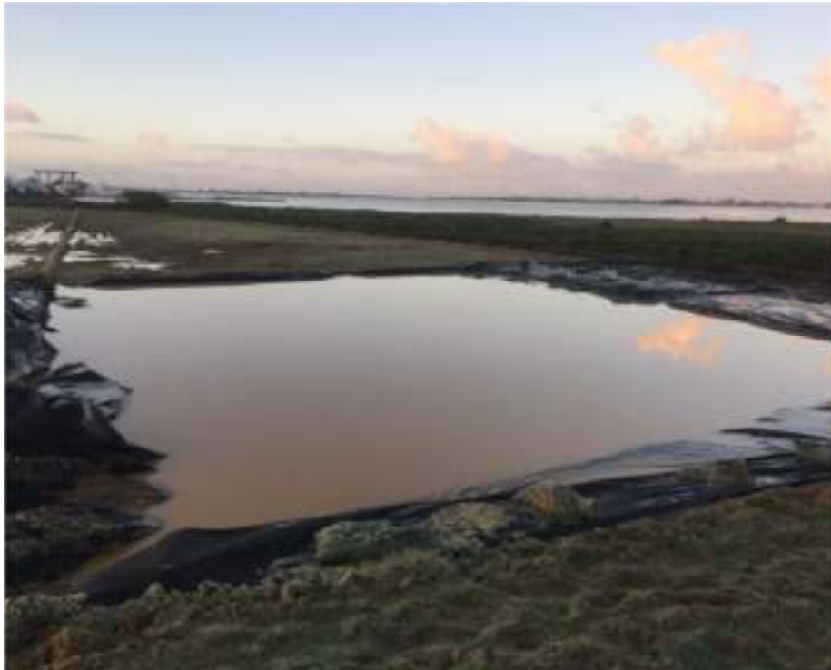
Installed BMP After Rain Event – Sediment Trap
