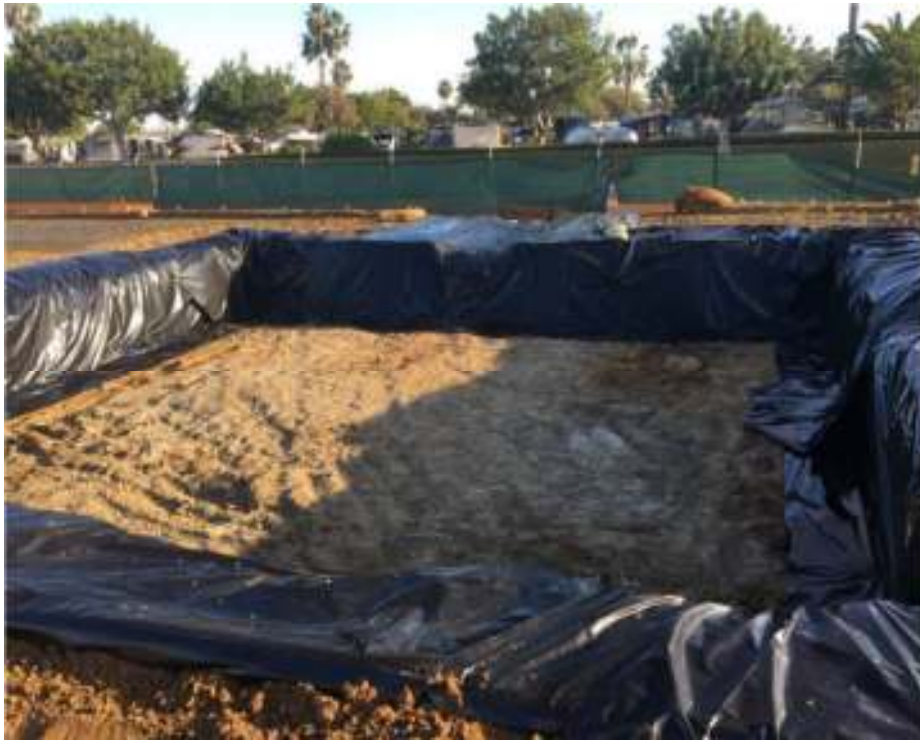
Installed BMP Before Rain Event – Sediment Trap
