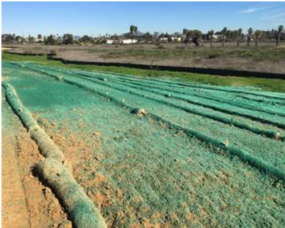
Installed BMP – Fiber Rolls and Bonded Fiber Matrix with Hydroseed
