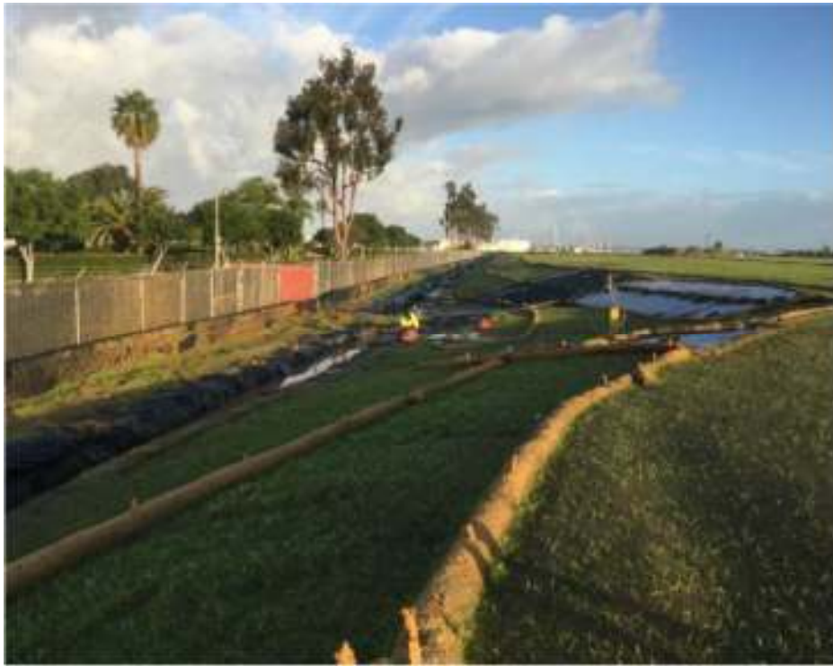
Installed BMP After Rain Event – Sediment Traps, Pumps, Fiber Rolls and Bonded Fiber Matrix with Hydroseed
