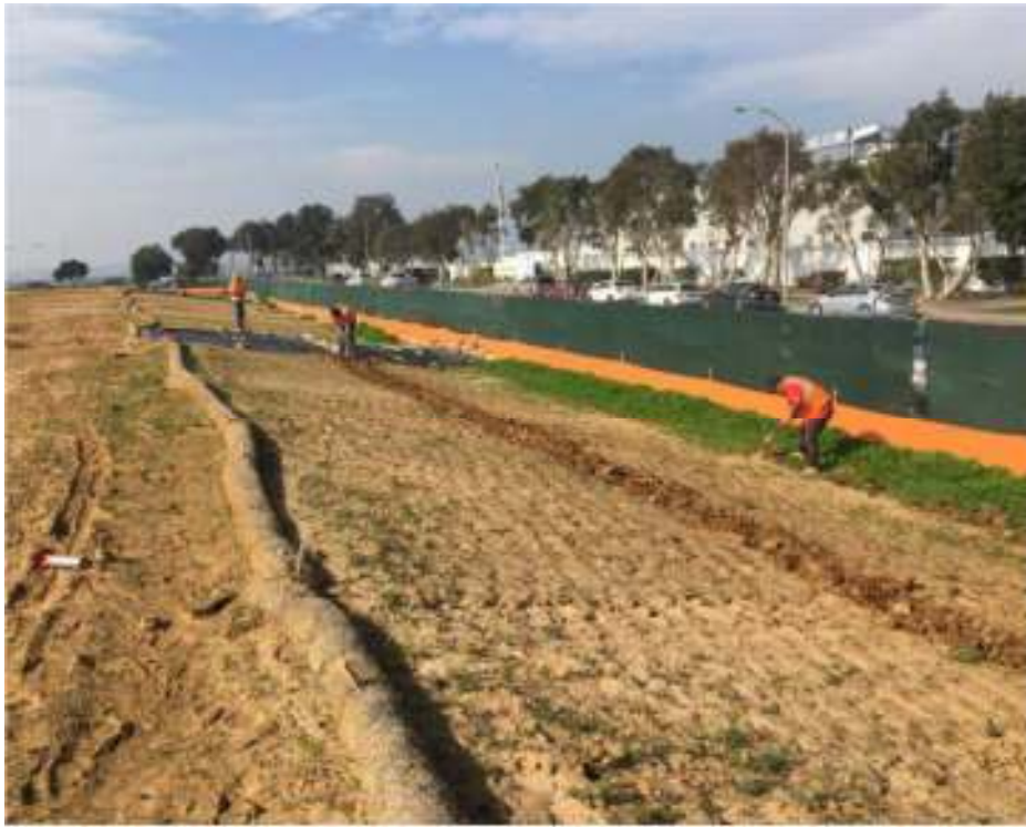
BMP Installation – Fiber Rolls
