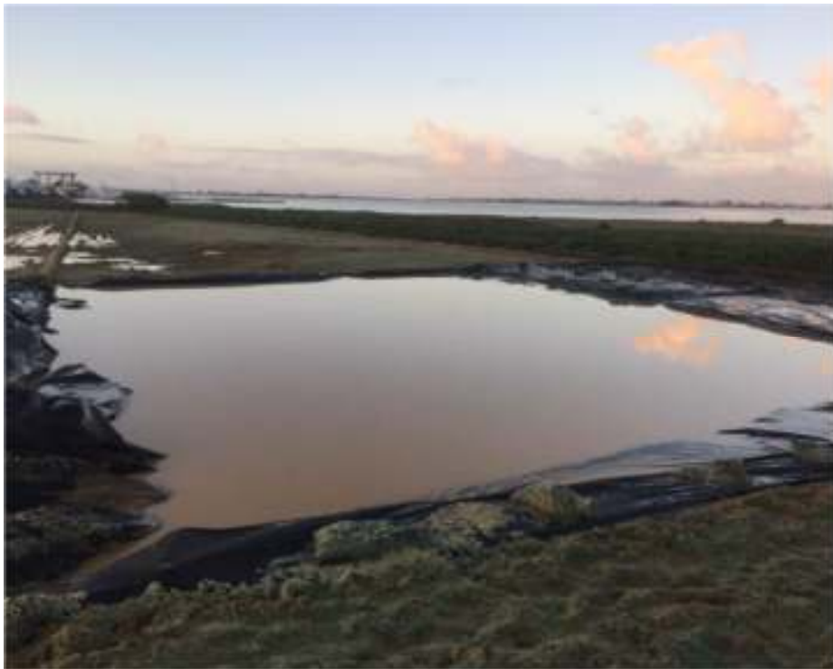
Installed BMP After Rain Event – Sediment Trap
