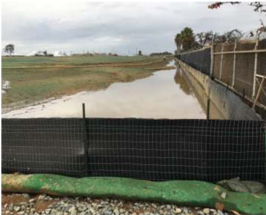
Installed BMP After Rain Event – Sediment Traps and Wire Backed Silt Fence
