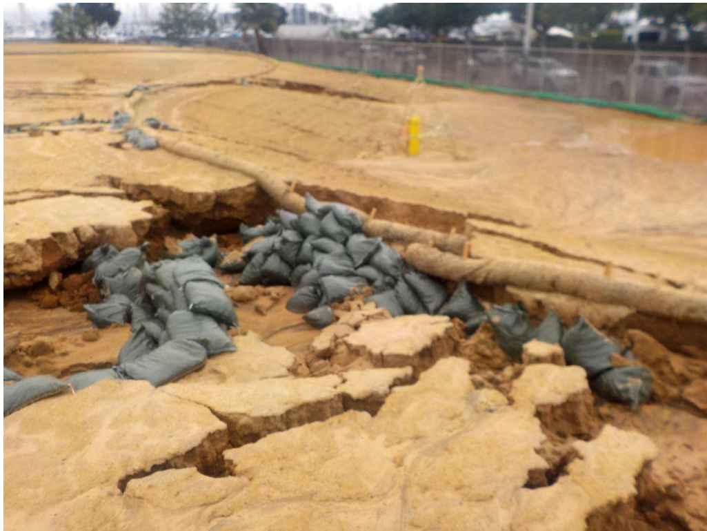
4. View of gravel bags deployed within erosion rill.
