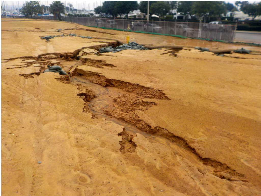
5. Upstream view of erosion rill and gravel bags within the erosion rill.
