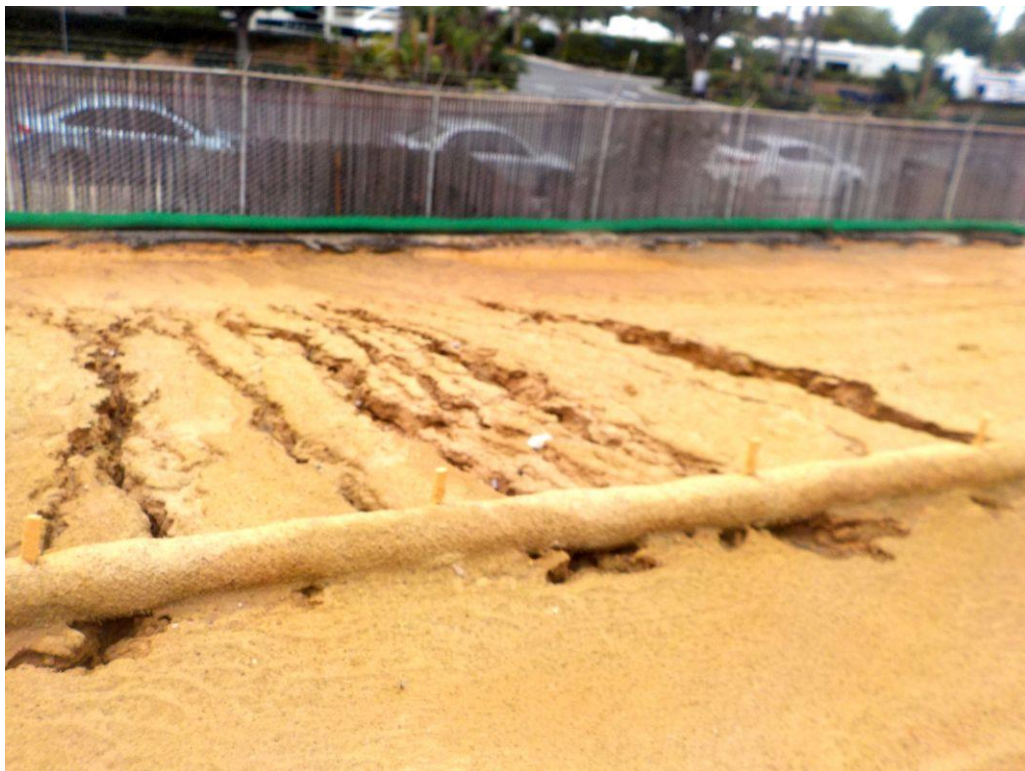
6. View of fiber roll at the top of slope along western perimeter.
