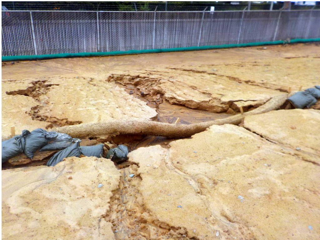
8. View of gravel bags and fiber roll at erosion rill along western perimeter of Site 3.
