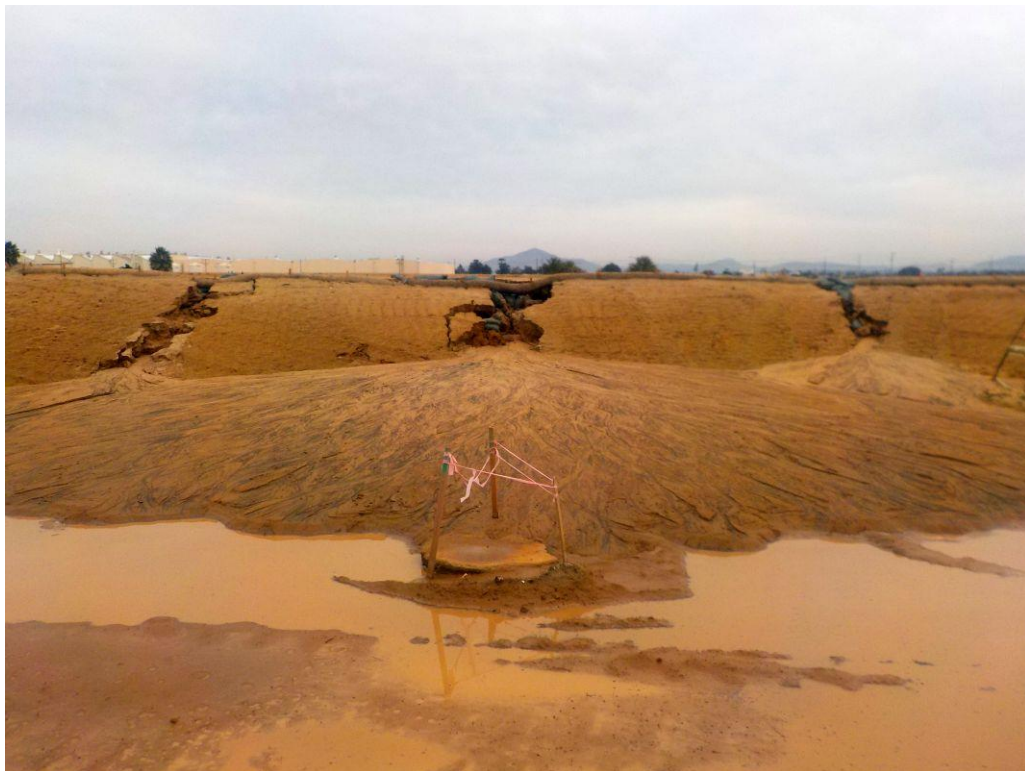
2. View of Site 3 erosion rills and sediment plumes along western perimeter.
