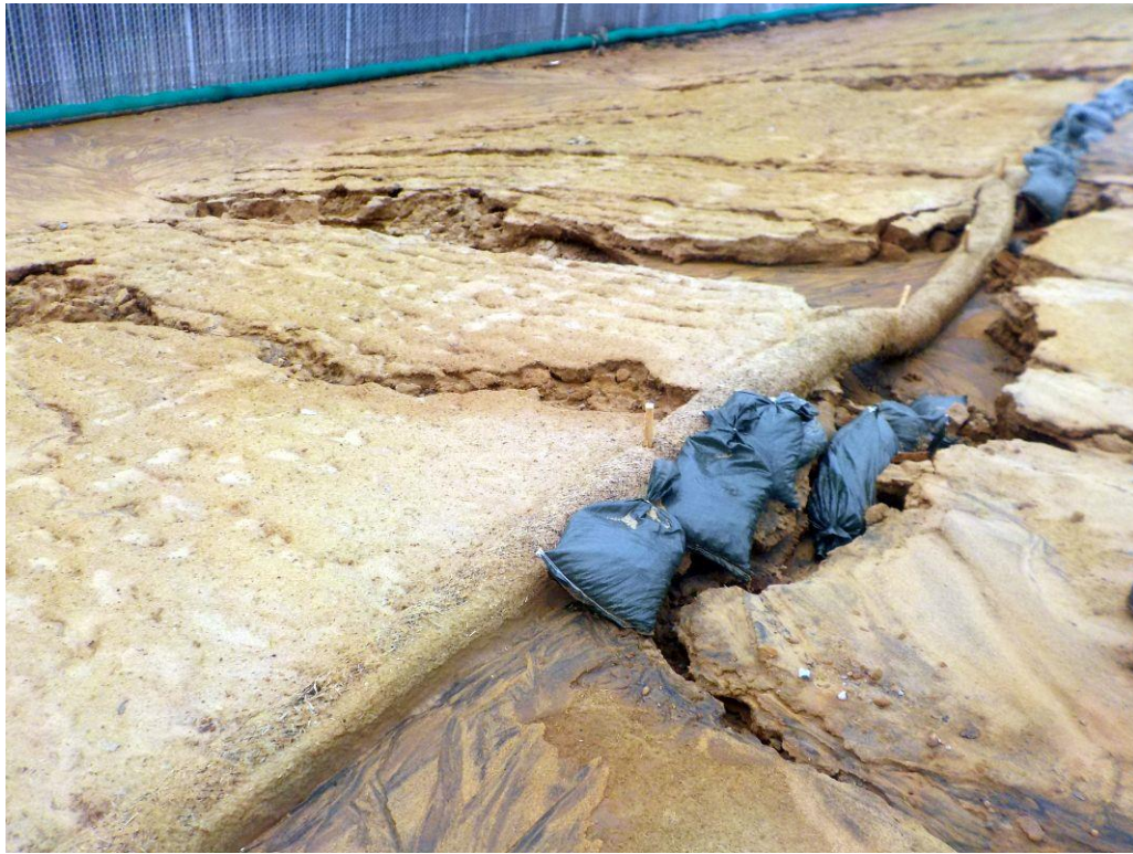
7. View of gravel bags and fiber roll at the top of slope along the western perimeter of Site 3.
