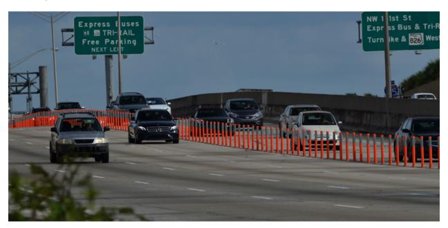
Candlestick traffic cones are installed in dense rows and are meant for temporary installations. Manufacturers state their products have a life span of one to two years.<sup>1</sup>
