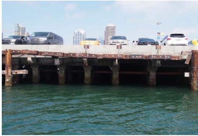
Missing fender piles
