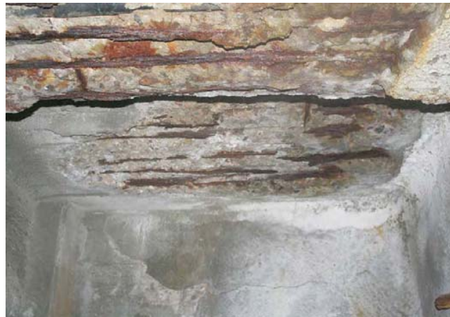
Severe corrosion of reinforcing steel
