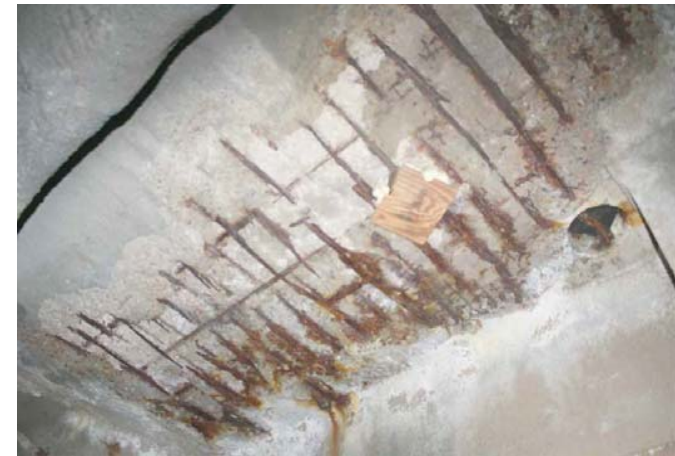
Major corrosion of reinforcing steel
