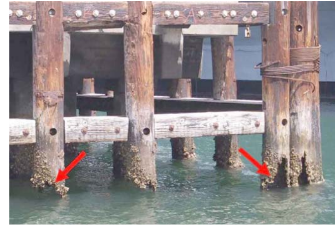
Rotten timber fender piles
