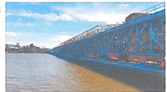
L & D 15 Service with Suspended Platform
