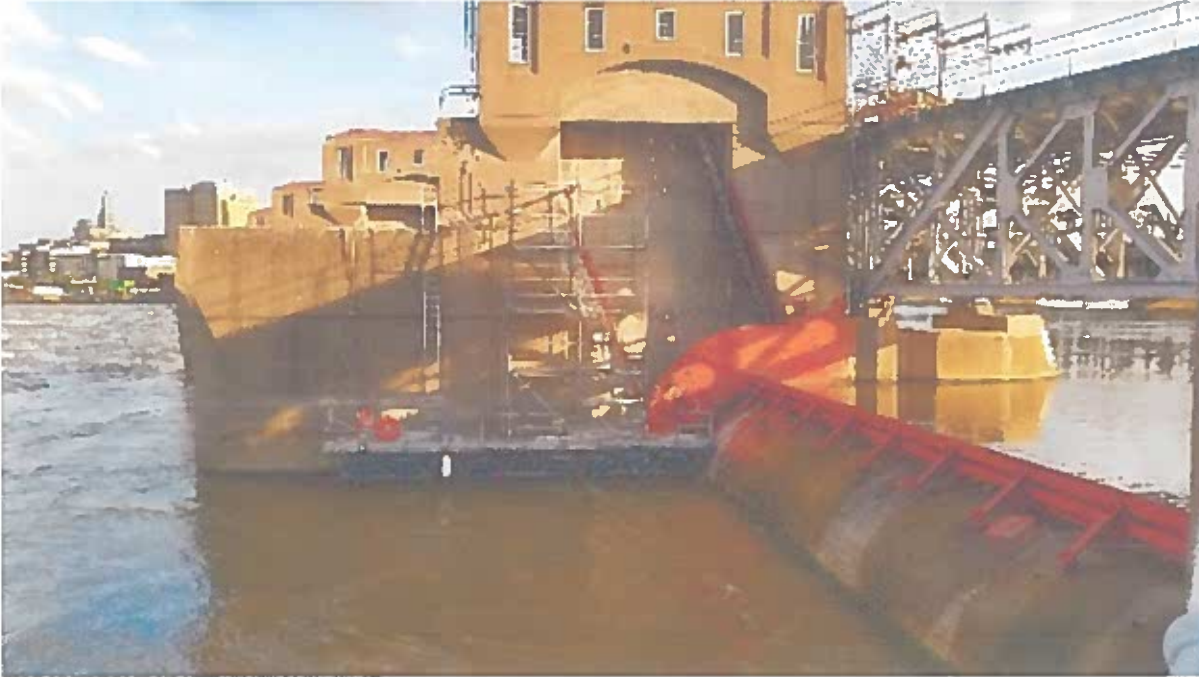
Work on Roller Gate Rack without use of a barge
