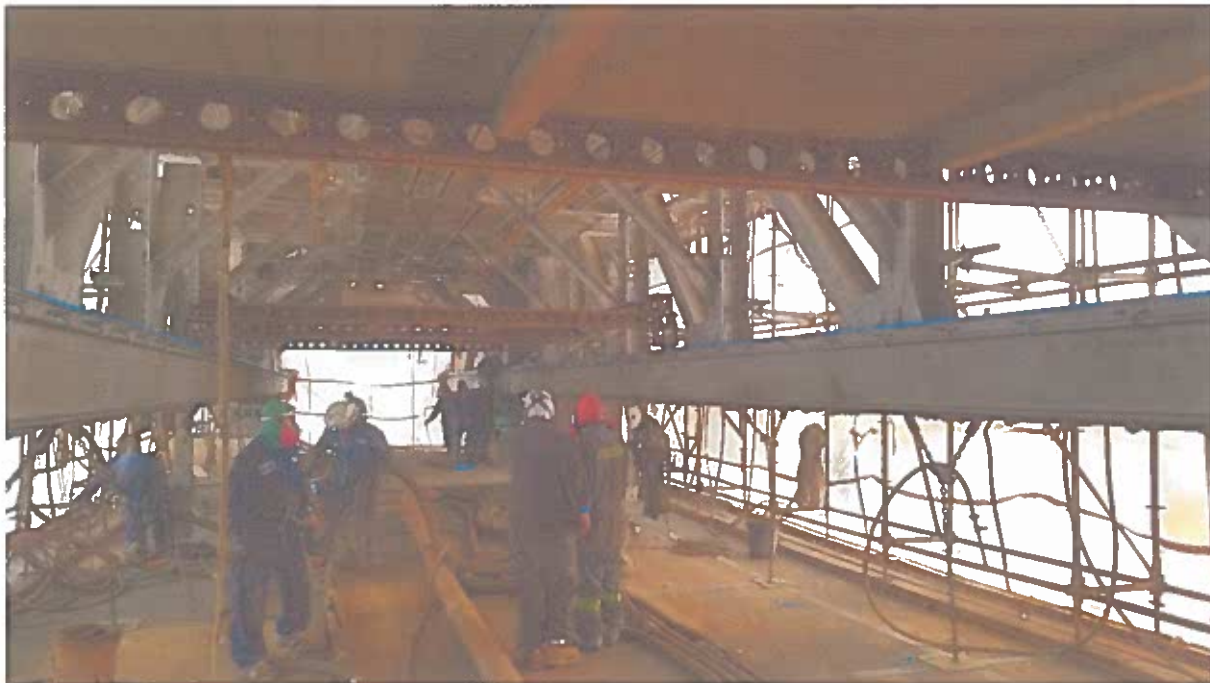
Inside Containment during abrasive blasting (hazardous/lead based paint) and coating operations
