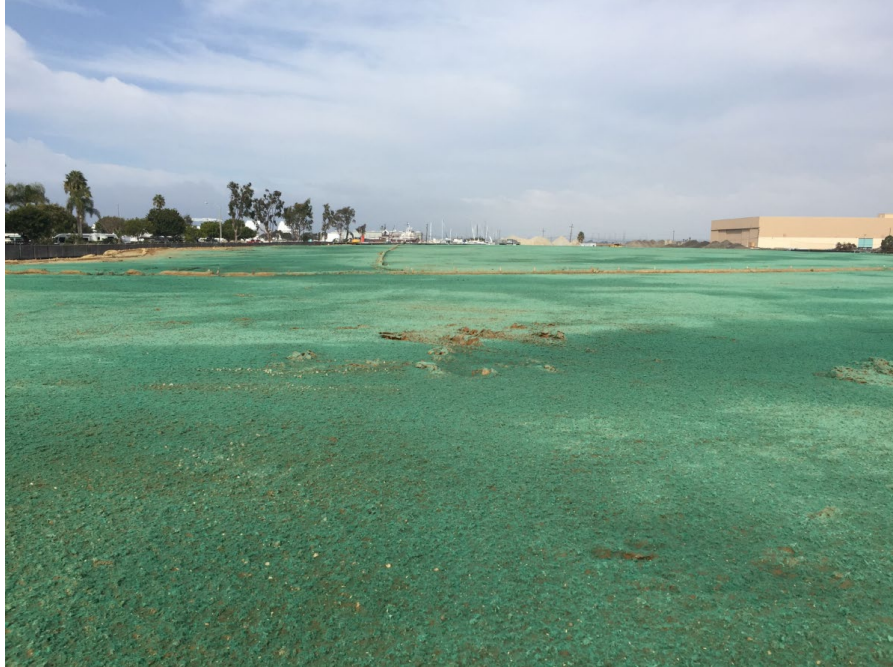
BMP Implemented – Bonded Fiber Mulch with Hydroseed Mix
