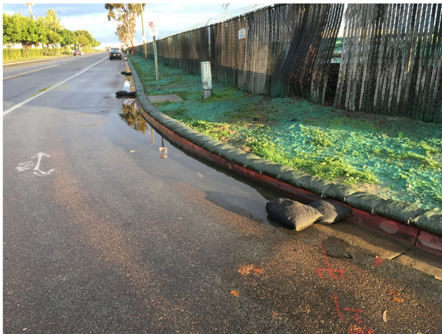
Storm Water Runoff Inlet after rain event
