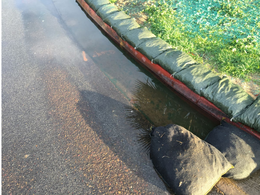
Storm Water Runoff Inlet after rain event
