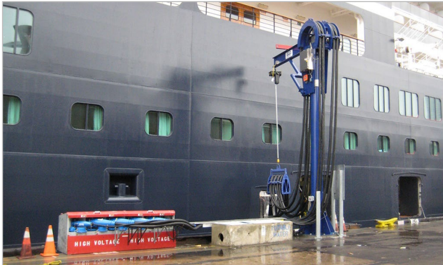
Figure IV.6-1 Street Cruise Ship Terminal Shore Power System 9
