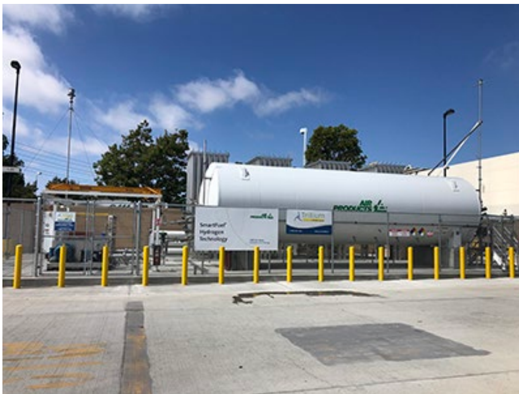
Figure 6-9. Orange County Transportation Authority 18,000-Gallon Liquid Hydrogen Storage Tank
